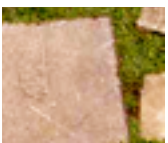
recycled concrete shows aggregate
