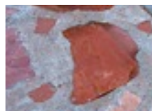
flat stone inlay in permanent concrete setting bed for walkway - consider patterns of bricks, coal blocks, cobbles, quartz rocks, and mineral samples
