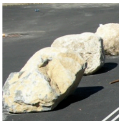
use of natural boulders (locally sourced from nearby site) to separate vehicles from schoolyard play areas
