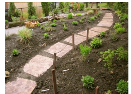
2'x2' concrete pavers stained mottled brown through a new urban meadow
