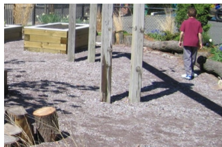
crusher run - a mixture of stone dust and aggregate
