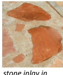
stone inlay in permanent concrete setting
