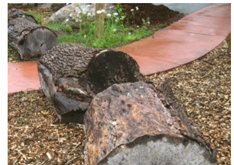
fibar (treated wood chips) a renewable and low cost walking surface / note the cast concrete walk with integral red color in background
