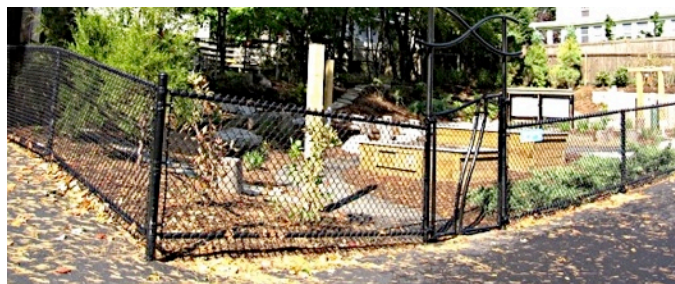
outdoor classroom - fully enclosed by black coated chain link fence (48" h) with custom entrance gateway (lockable)
