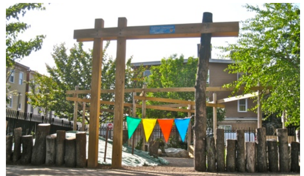
entrance gate - natural log pole with machine milled wood (within a locked schoolyard) flags denote OC / SY boundary (w/ log boundary fence)
