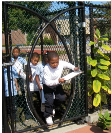
seedpod gate: child scale 5'-2" high opening, gate swings open for full access (w/secondary lockable gate)
