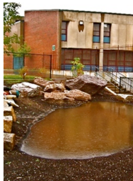
Rain garden, with schoolyard runoff (during construction)
