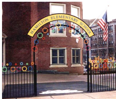
custom welded and painted steel gateway added to existing fence
