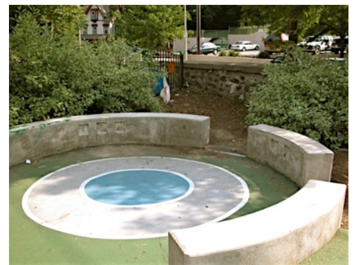
small amphitheater, meeting area, cast concrete with insert places for artwork tiles
